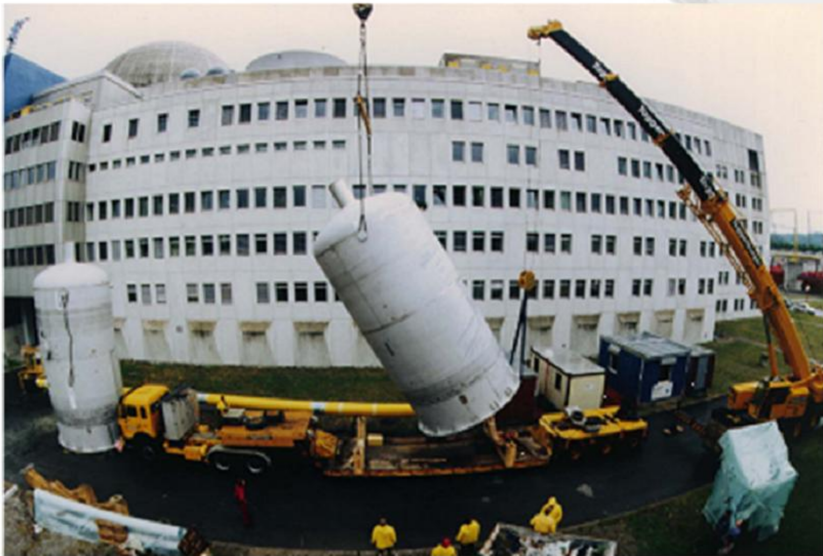
Delivery of two filter vessels to the NPP Leibstadt
