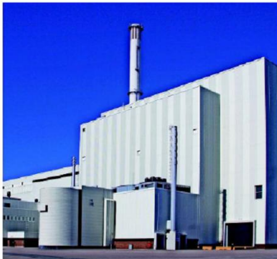
FILTRA/MVSS (cylindrical building shown at the lower left corner) at Forsmark 3, Sweden. Photo: Hans Blomberg.
