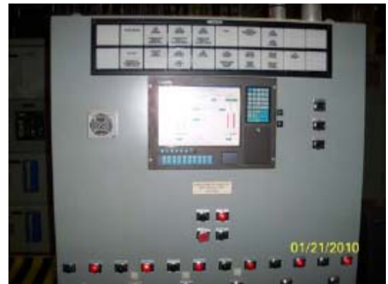
Fig.5.23 Hydrogen Water Chemistry Controls
