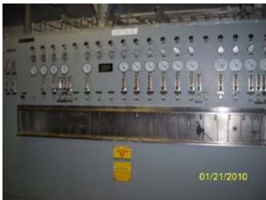
Fig.5.24 Chemistry sample Panel
