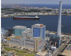
Isogo Thermal Power Plant
