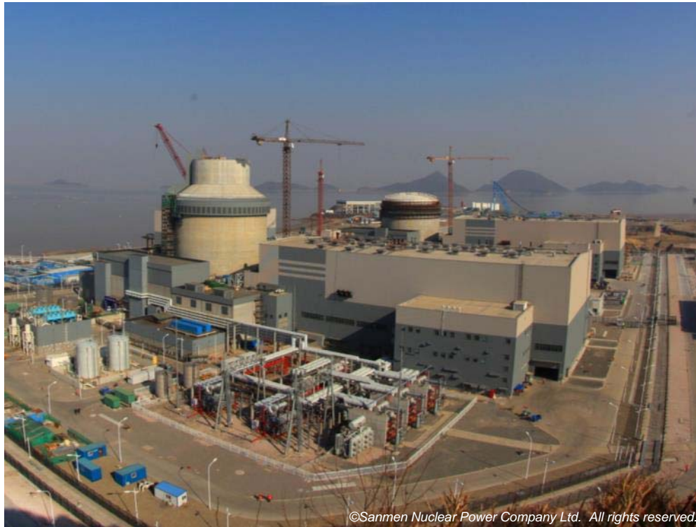
AP1000 Plant Site at Sanmen, China
