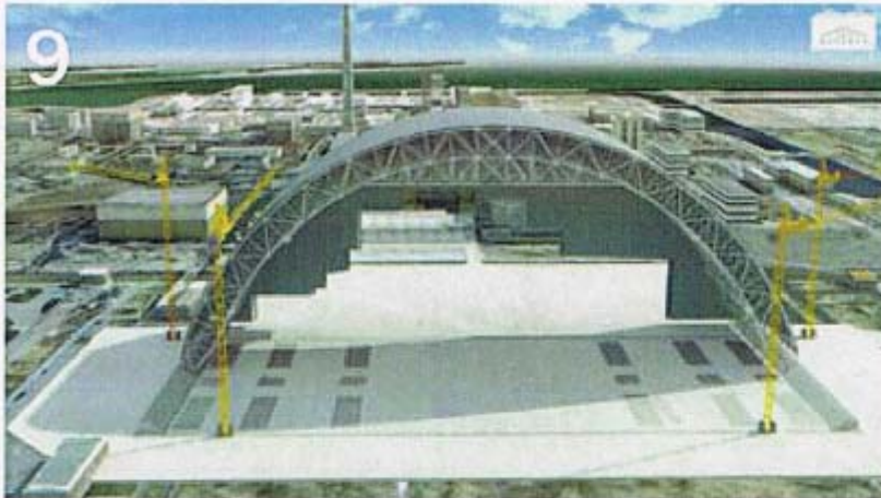
End wall installed and first section moved into holding area
